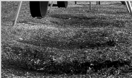
Playground with loose fill material ALWAYS ends up with "dished out" areas at critical fall locations.
